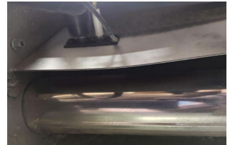
Fourneau rampe gaz
